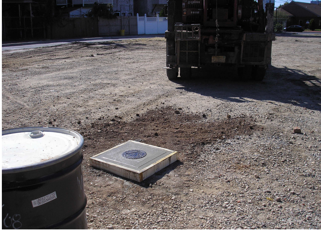
PHOTO 5: View of MW-4 Reconstructed.
