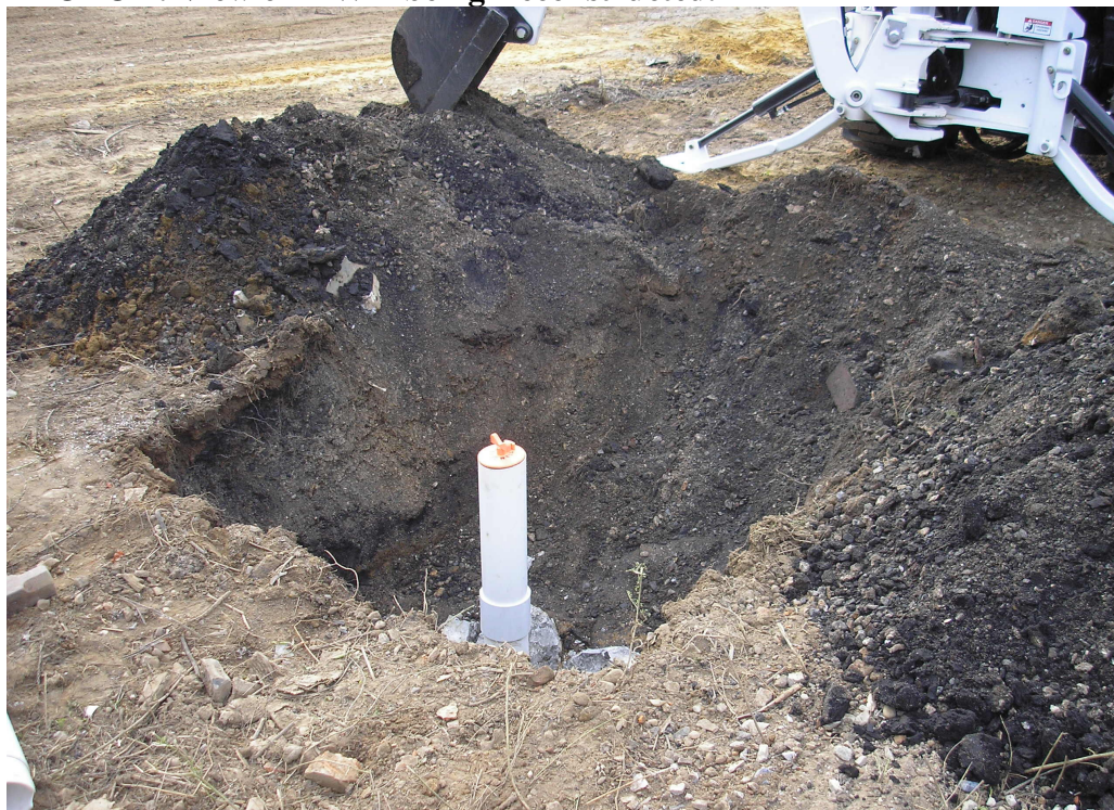
PHOTO 1: View of MW-1 being Reconstructed.
