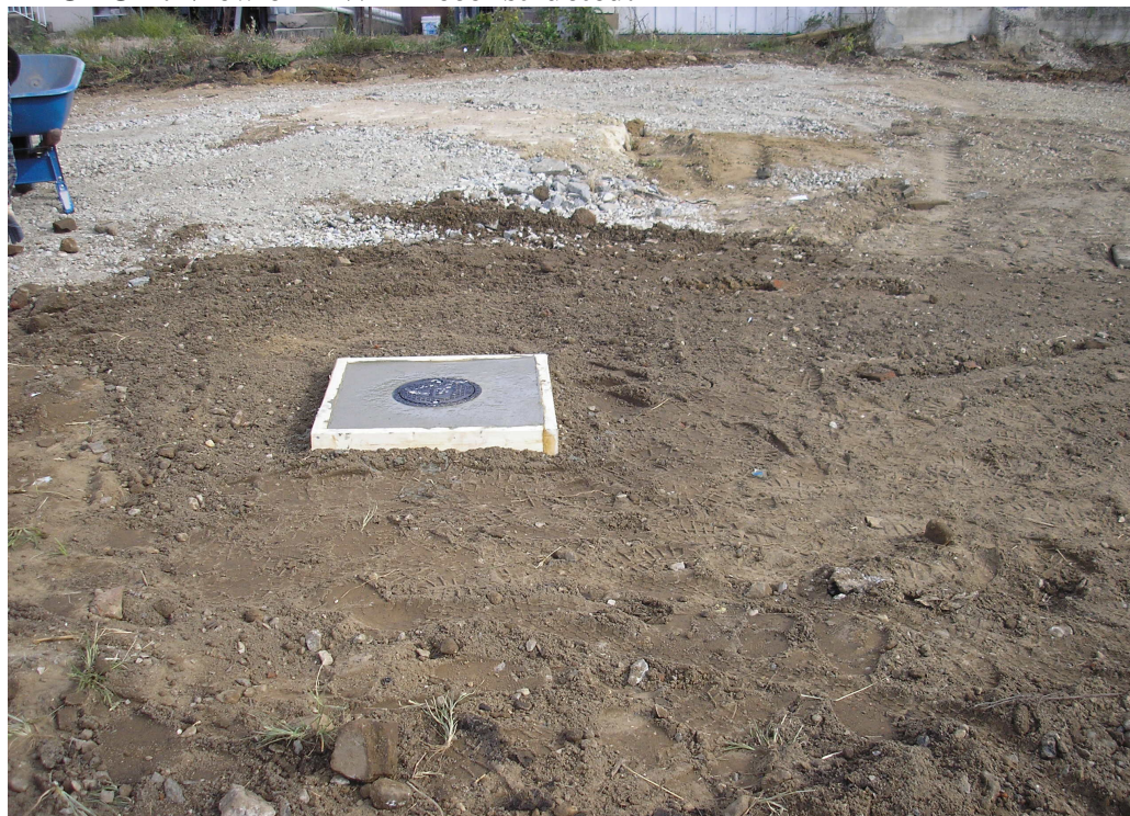
PHOTO 2: View of MW-1 Reconstructed.
