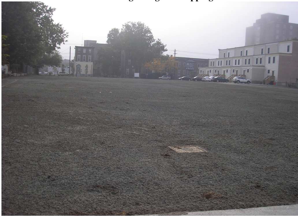
PHOTO 8: View of Site after Regrading and Capping.
